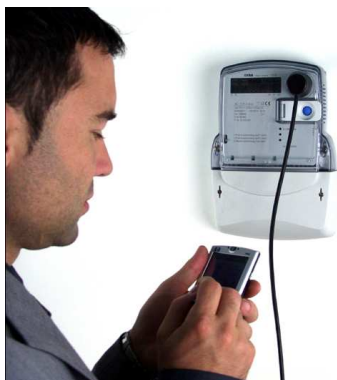
Fig. 28: Meter readout via an IR optical interface
